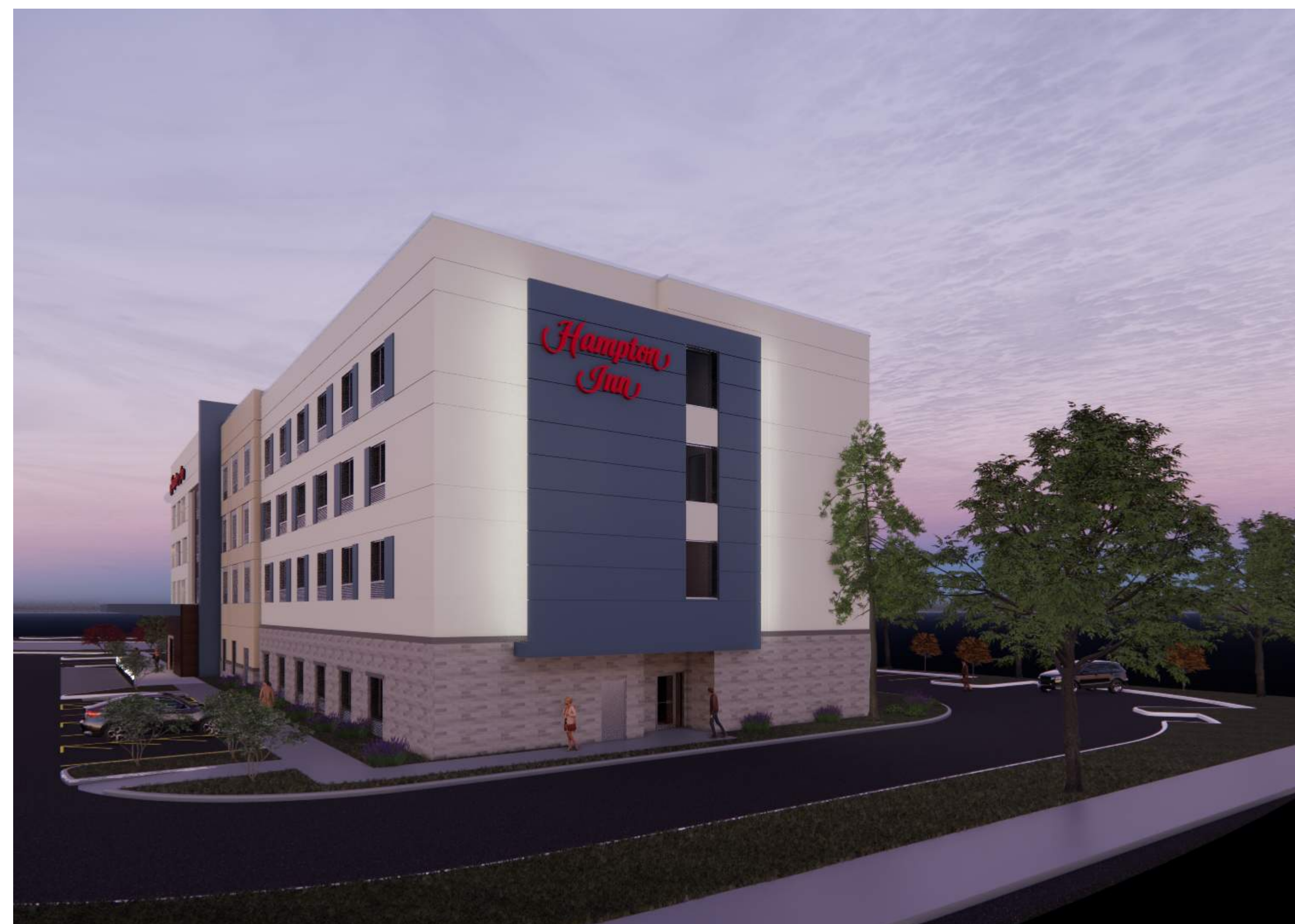
VIEW 3 - SE CORNER
