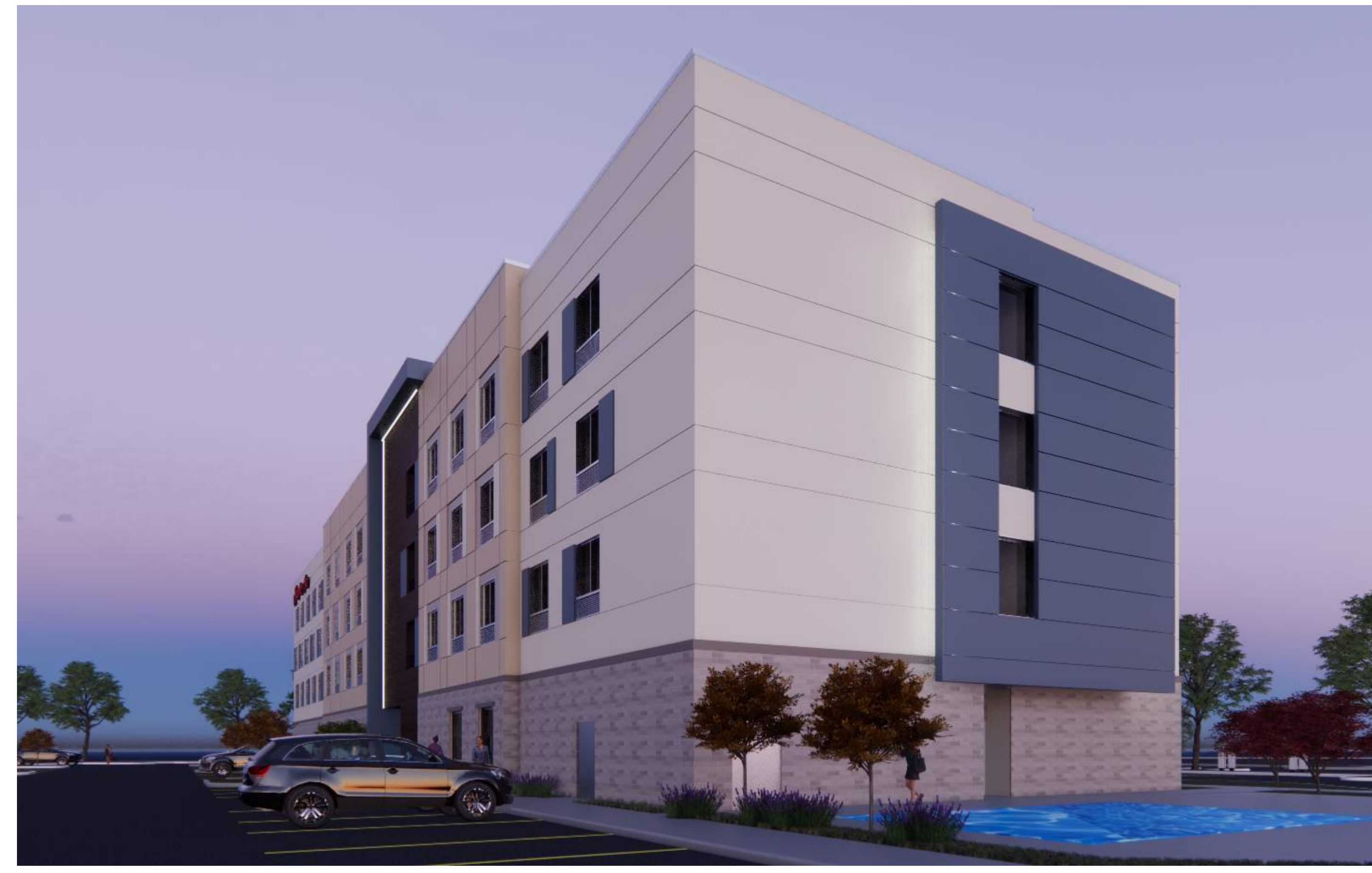
VIEW 6 - NW CORNER
