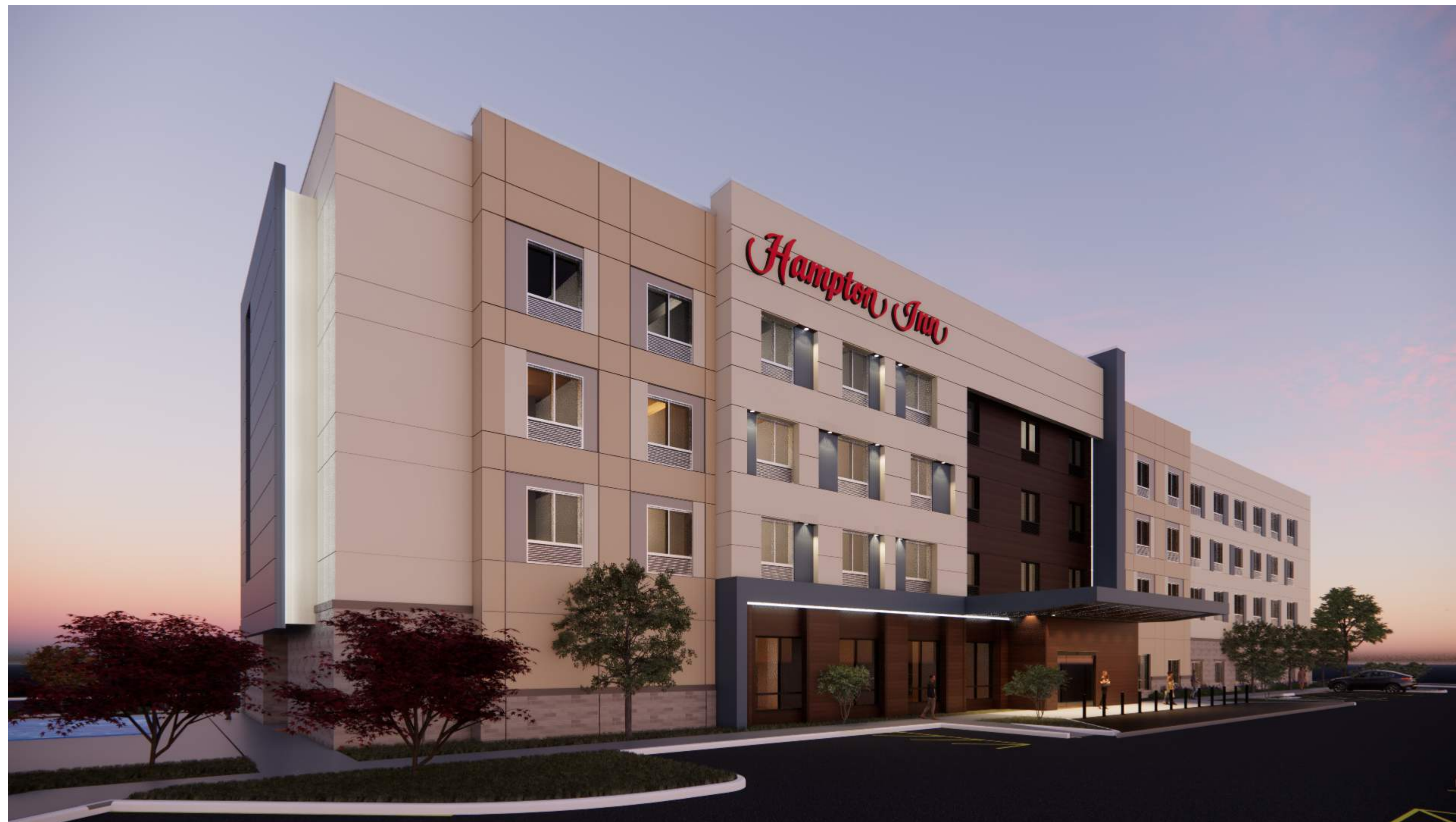
VIEW 1 - SOUTH FACADE
